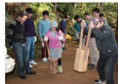
A tool called a rammer is used to pack in soil
