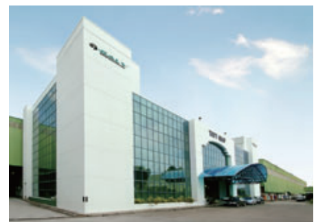
Appearance of the exterior
