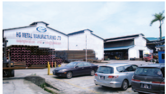
Eversendai Corporation Bhd in Malaysia (top) HG Metal Manufacturing Limited in Singapore (bottom)
