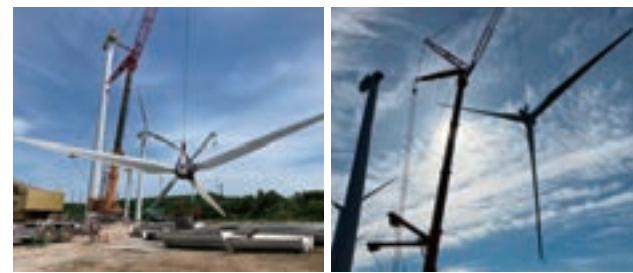
Dismantling wind turbines
