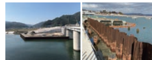
We delivered steel sheet piles needed at the bay construction sites along the Sanriku Coast, which was damaged by the Great East Japan Earthquake, and reused ones that were still valuable after use.
