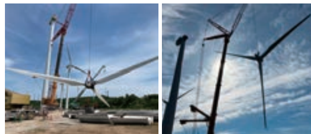
Dismantling wind turbines
