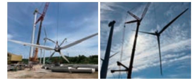
Dismantling wind turbines
