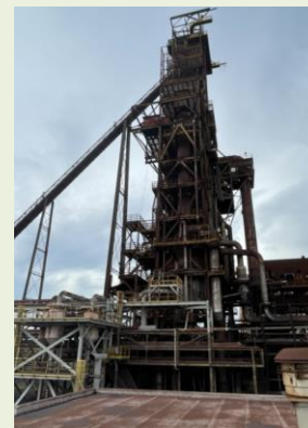
The HBI producing Shaft
